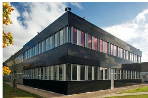
Fig.1 ZERO2020 BUILDING RETROFIT TEST-BED IN CORK INSTITUTE OF TECHNOLOGY, IRELAND
