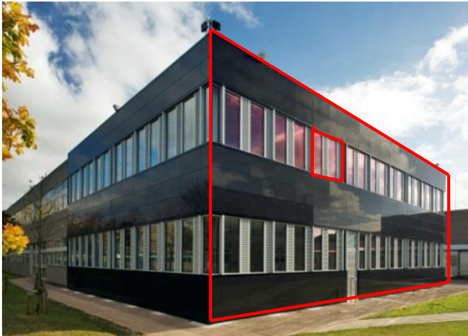
Retrofit Space External
