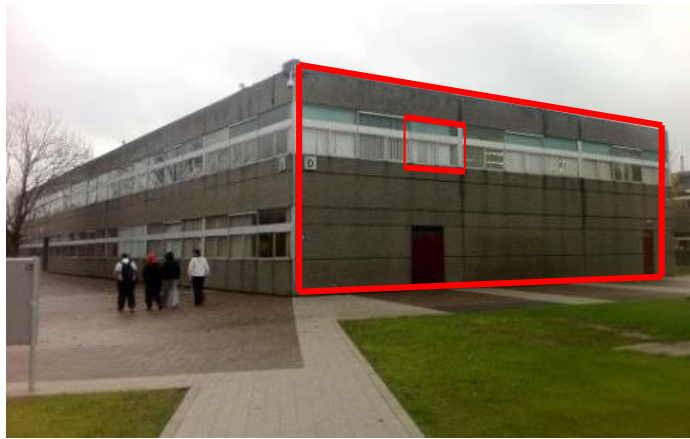
External West Facing First Floor Zone
