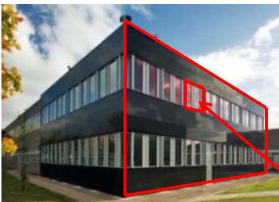
west facing retrofit test space
